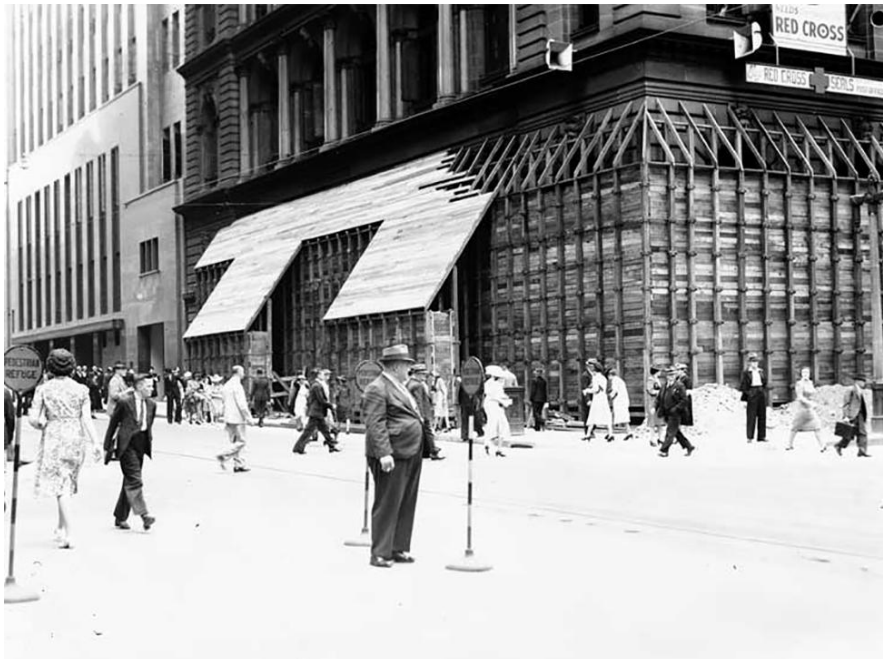
Air raid protection erected around the old Sydney General Post Office on the corner of Pitt Street and Martin Place in 1942. The new post office building is also visible on the left as are Red Cross posters on the GPO and signs for a pedestrian refuge in the street. Source: National Archives of Australia.
